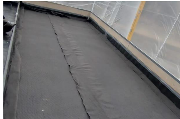
Fig. 6 Drain and filter, planar geodrain
